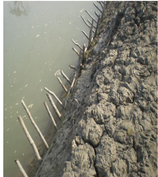
(f) Local protection of embankment with illegally harvested timbers
