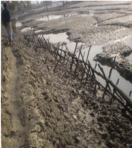
(f) Local protection of embankment with illegally harvested timbers
