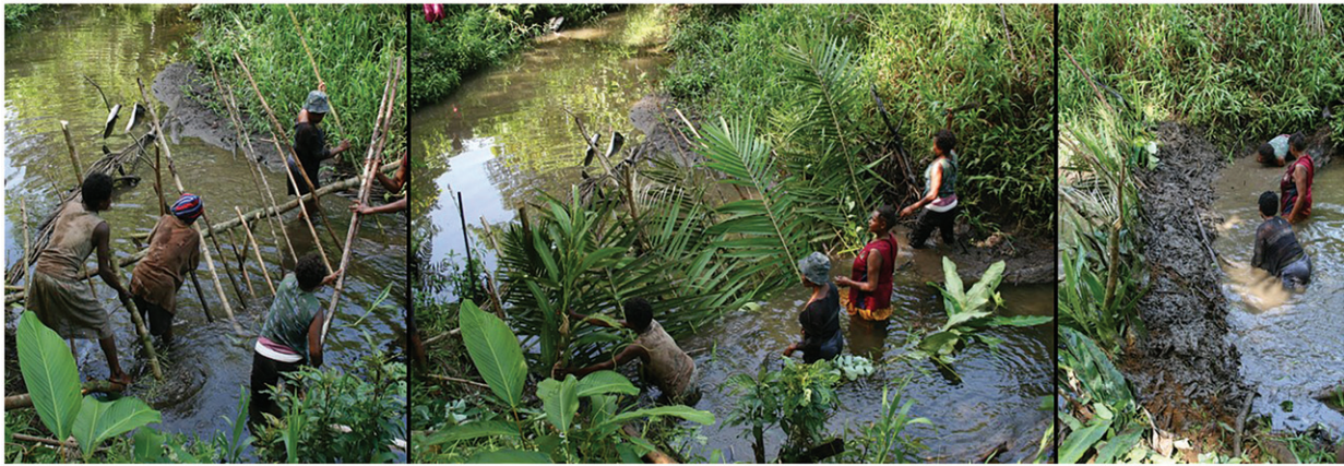
Figure 3. Weir construction (photographs: Lara Lamb).
