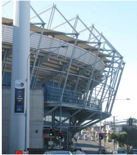
Figure 5-12: The Gabba Stadium on Stanley Street overhanging Stanley Street
