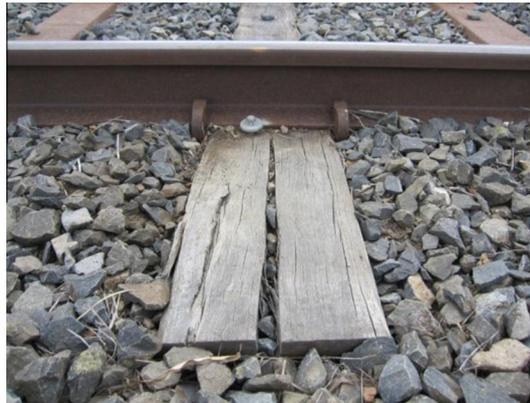
Fig. 3. End splitting of timber sleeper.
