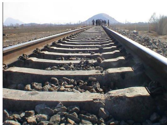
**Fig. 9.** Derailment failure of concrete sleepers [27].
