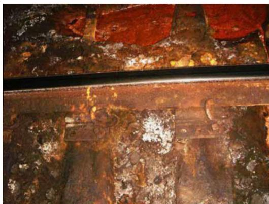
Fig. 20. Corrosion in steel sleeper [50].
