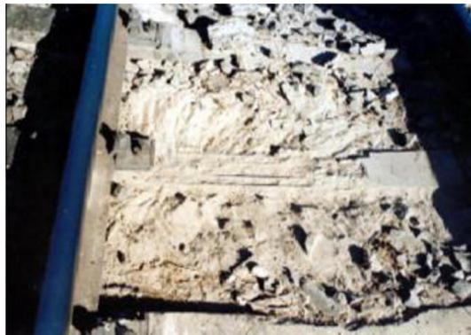
Fig. 18. Failure of concrete sleeper as result of bar corrosion [47].
