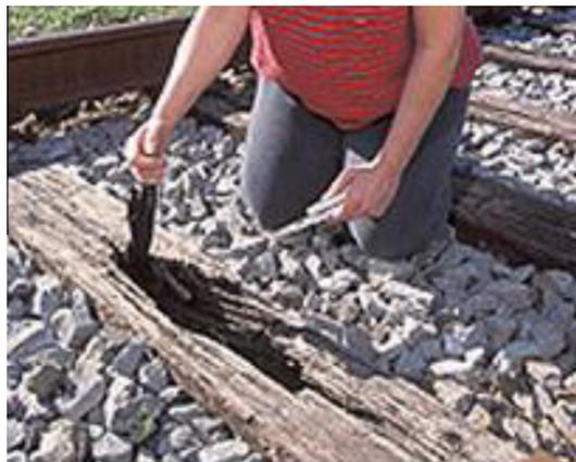
Fig. 4. Termite attacks in timber sleeper [14].
