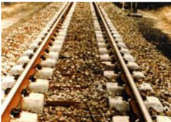
(a) twin-block reinforced concrete
