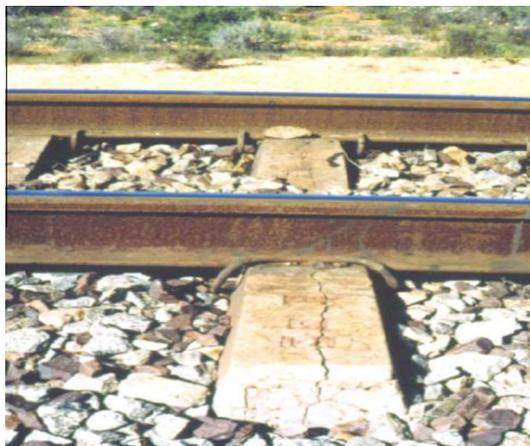
Fig. 16. Cracking in concrete sleeper due to AAR [44].
