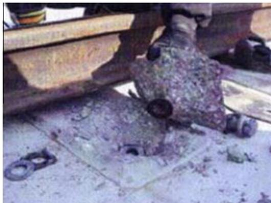
Fig. 19. Conical crack due to ice forming in slab track [48].
