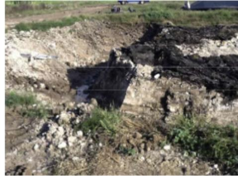
Fig. 3. Section of crust removed from an anaerobic lagoon by an excavator after desludging indicating crust thickness [12].
