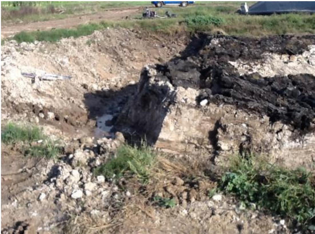
*Figure 3: Section of crust removed from an anaerobic lagoon by an excavator after desludging indicating crust thickness (McCabe et al. 2013).*
