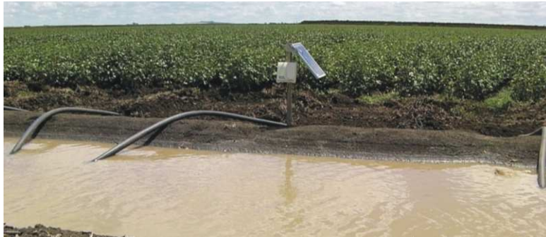
Surface irrigation system
