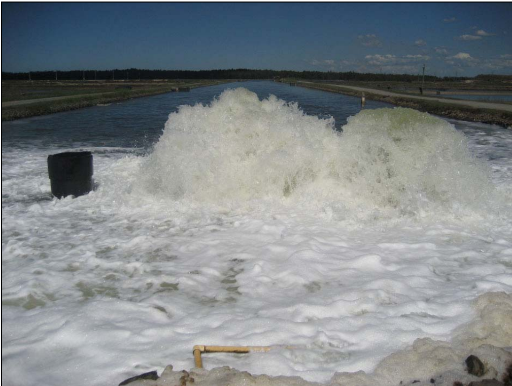
The main river pumps for the farm.
