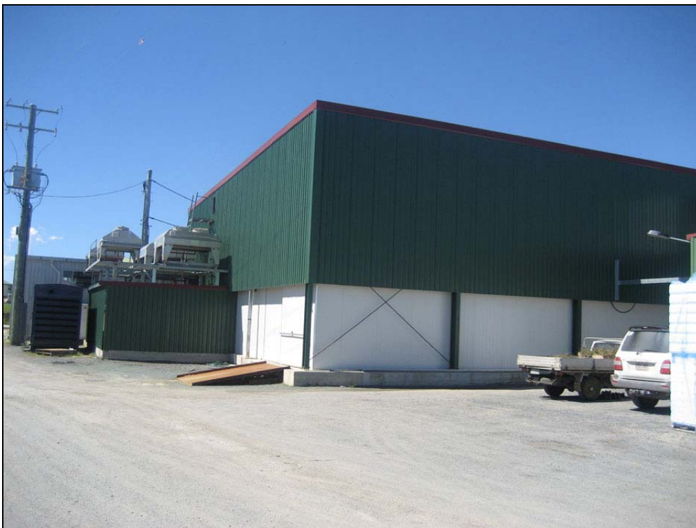
The Main Freezer Shed
