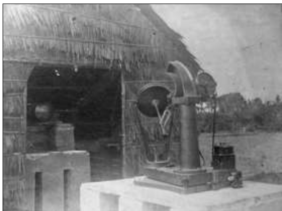
Figure 20 (left): A close-up of the siderostat and drive (courtesy: Schuster Papers and Photographs Archive, Royal Astronomical Society).
