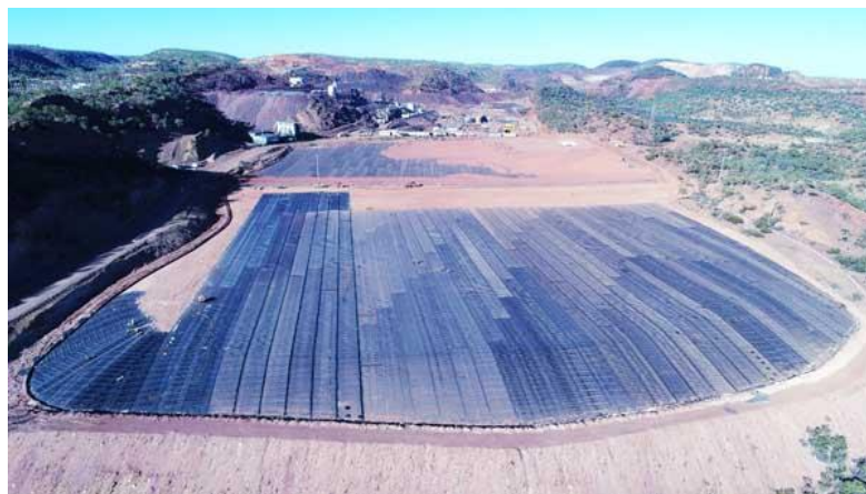
Figure 128: Mine waste cover in a tailings pond at Capricorn Copper (Australia), (2019)
