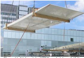
Figure 11. Lightweight GFRP sandwich roof [24]
