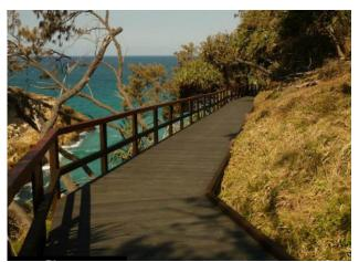
Figure 6. Composite sandwich boardwalks.
