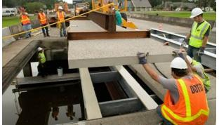
Figure 4. Balsa-cored composite bridge deck [13].
