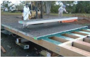
Figure 8. FRP sandwich bridge beams at USQ.
