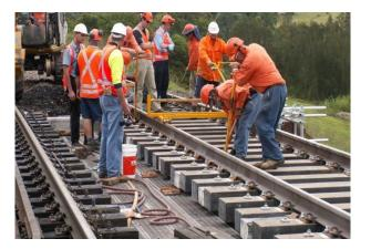
Figure 13. Composite sandwich railway sleepers
