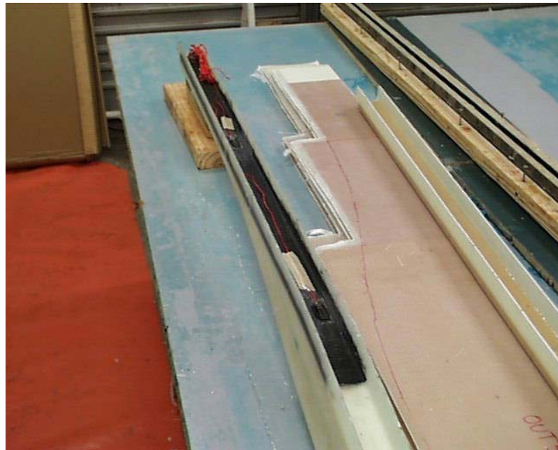
Figure E.8 Carbon Reinforcement Laminated to Inner Floor
