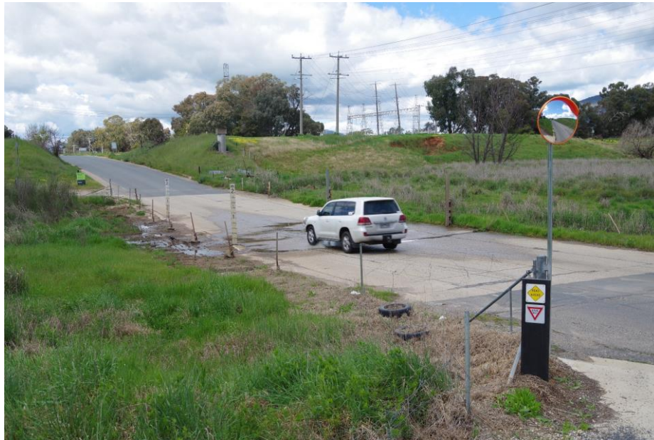
Figure 2.1. Typical floodway implemented on a rural road.
