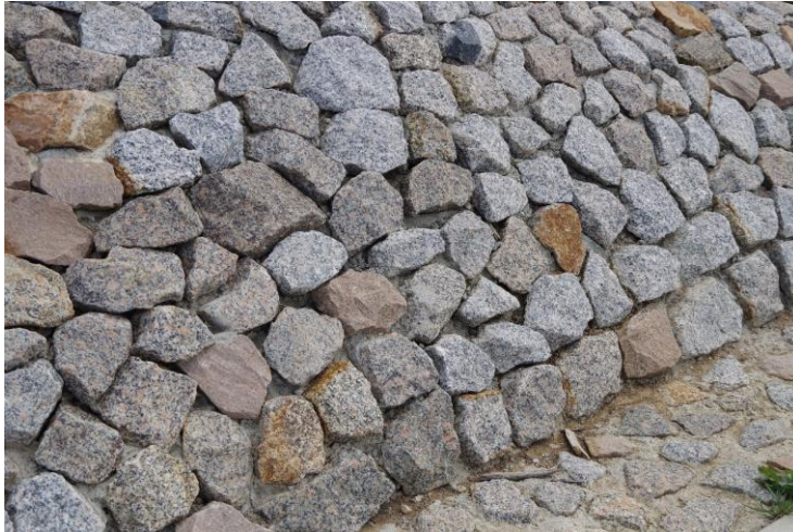
Figure 3.32. Typical rock pitching with concrete protection.
