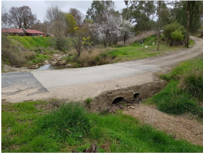
Figure 3.11. A typical raised floodway construction.
