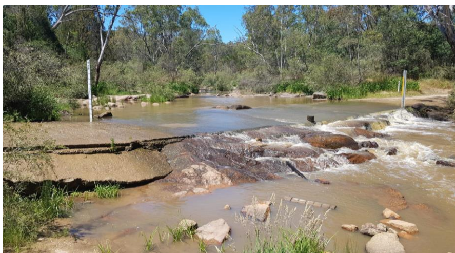
Figure 1. A typical concrete floodway structure.
