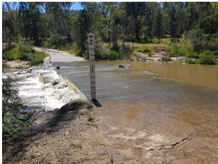
Figure 3.10. A typical level floodway construction.
