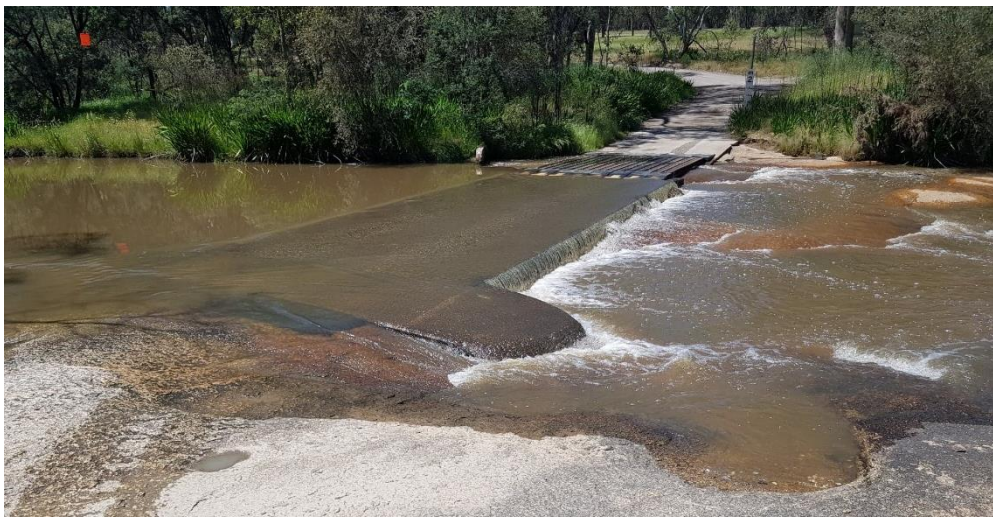
FIGURE 1. A typical low-water floodway crossing structure situated in a perennial waterway.
