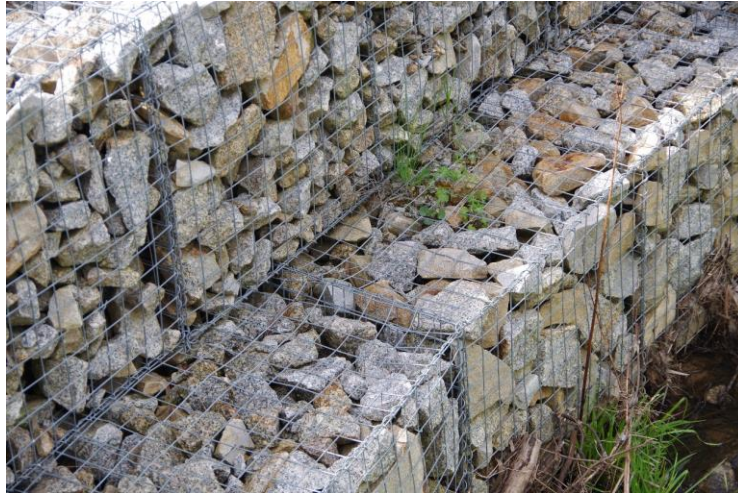
Figure 3.30. Typical gabion rock basket protection.
