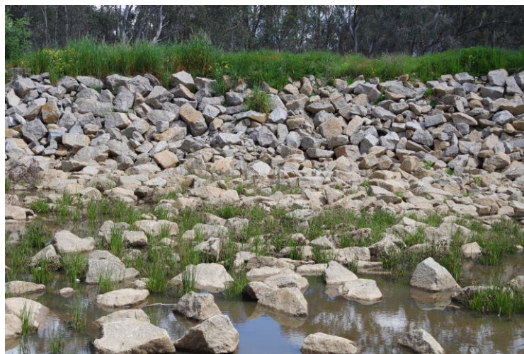
Figure 3.29. Typical dumped rock riprap protection.
