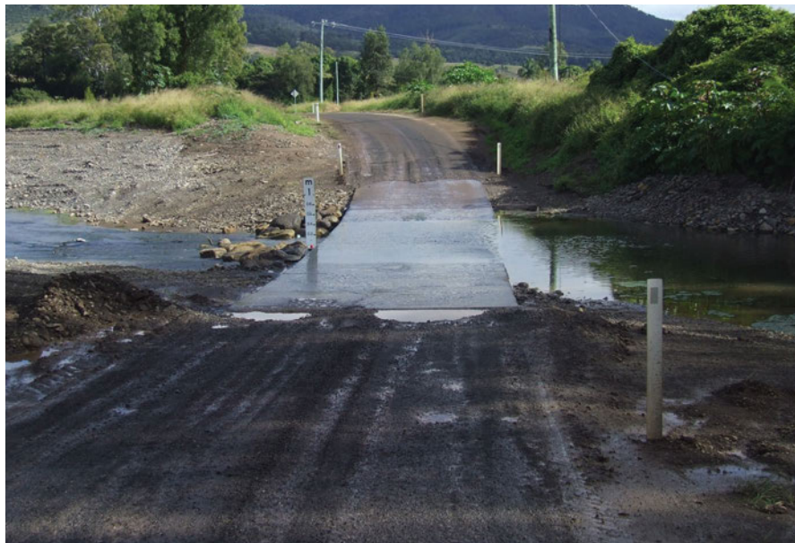
Figure 1. Floodway structure implemented in a low flow watercourse (Lockyer Valley Regional Council, personal photograph, 16 June 2011).
