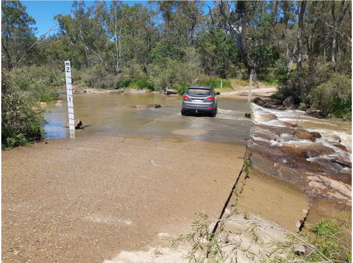
Figure 1.1: A typical rural concrete floodway.
