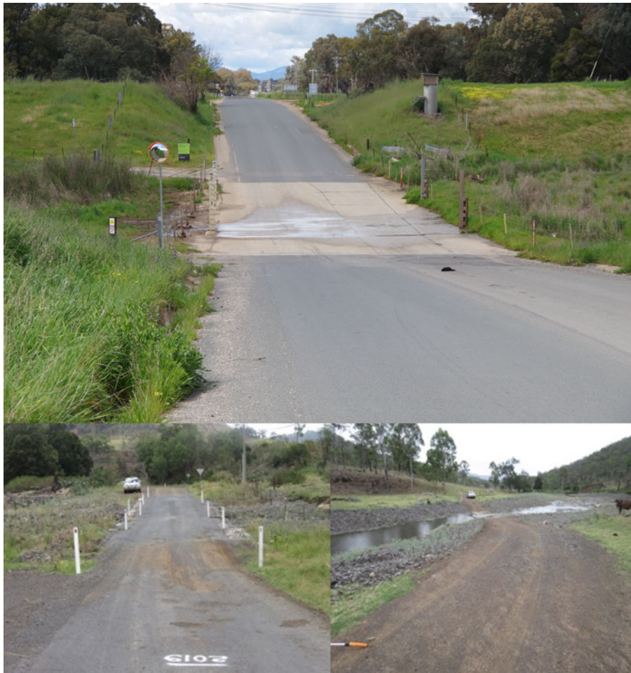
Figure 2.2: Typical floodway types (Lockyer Valley Regional Council, 2013).
