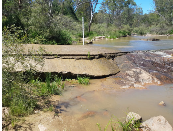
Figure 2.5: Undermined structure due to erosion.
