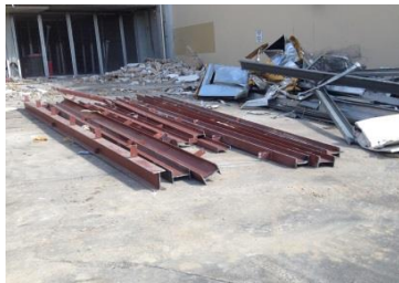
Figure 4.6: Steel elements from demolition in Toowong, Australia Source: Author (2015).
