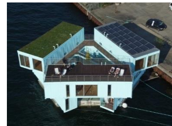
Figure 4.8: Floating shipping container apartments in Denmark Source: Stella (2016).
