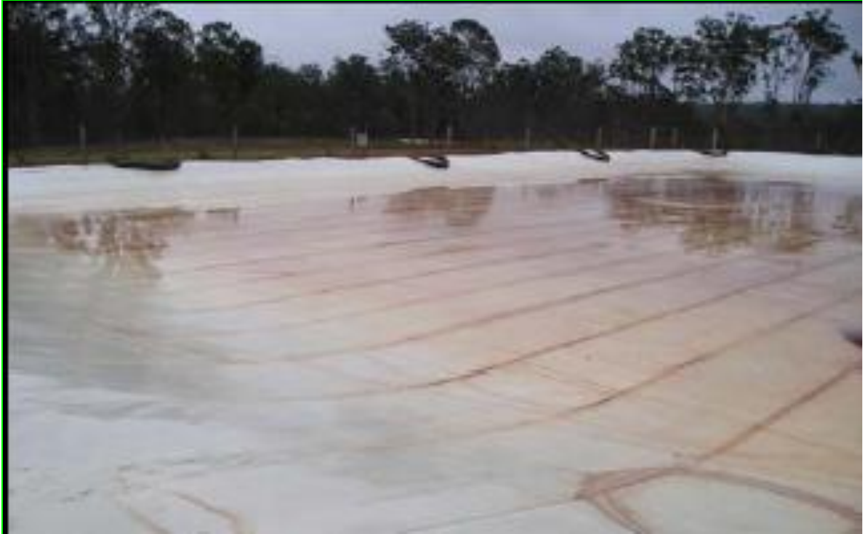
Figure 17: E-VapCap is a floating cover constructed as a single piece with holes spread evenly over the surface to allow rain to enter the storage.
