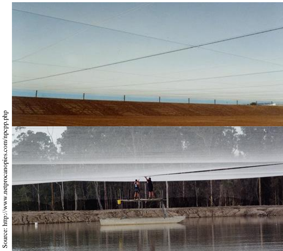
Figure 18: Netpro shade cloth is suspended above the surface of the water using poles and high tension cable.
