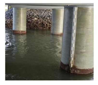
Figure 7.1. Novel FRP jacket utilisation in actual repair project
