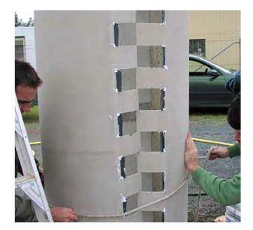
Fig. 9. GFRP composite pile repair system [70].
