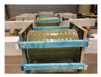
Fig. 7. Installation of GFRP jackets over the beams.
