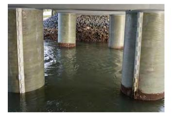
Fig. 17. Bridge piles repaired with FRP jacket [166].
