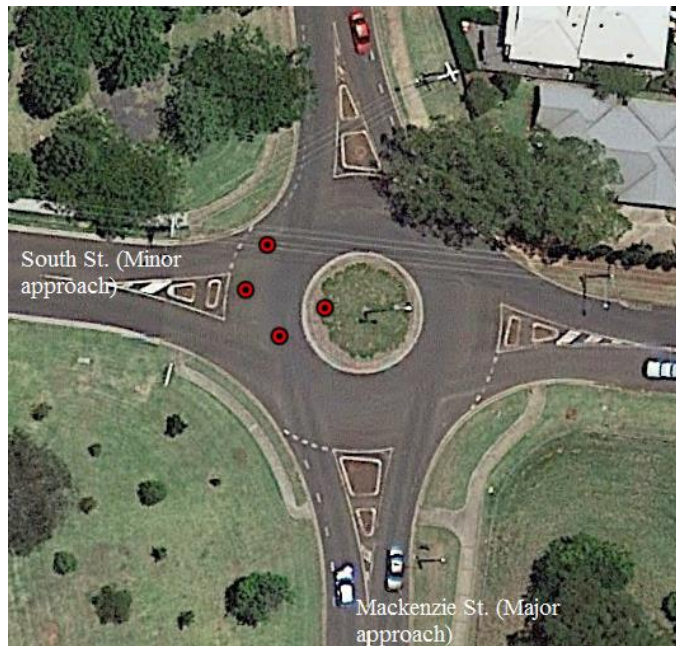
Figure 5.24 Roundabout R_SE13 between Mackenzie Street and South Street (Source: Aerial Image from Google Earth pro)
