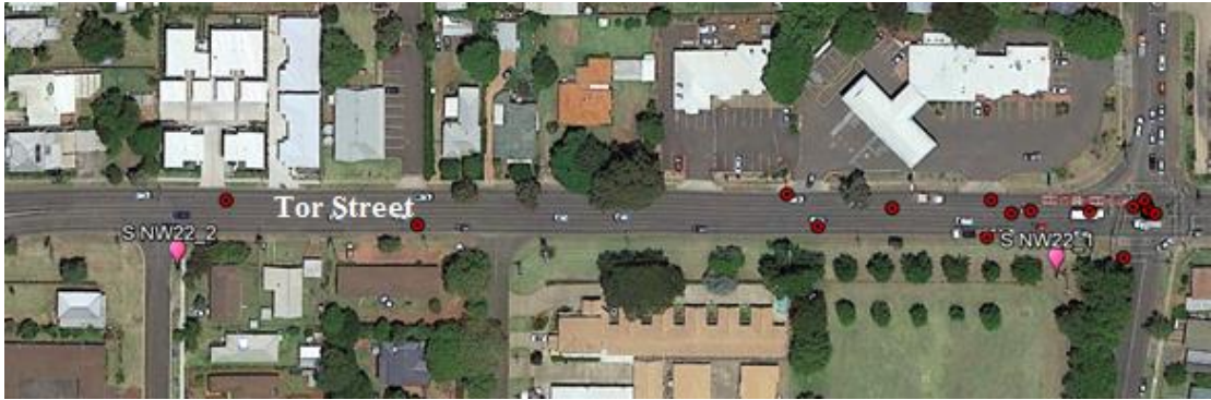
Figure 6.11 Segment S_NW22 on Tor Street (Source: Aerial Image from Google Earth pro)
