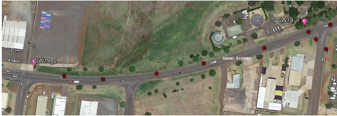
Figure 6.19 Segment S_SW19 on Anzac Avenue (Source: Aerial Image from Google Earth pro)
