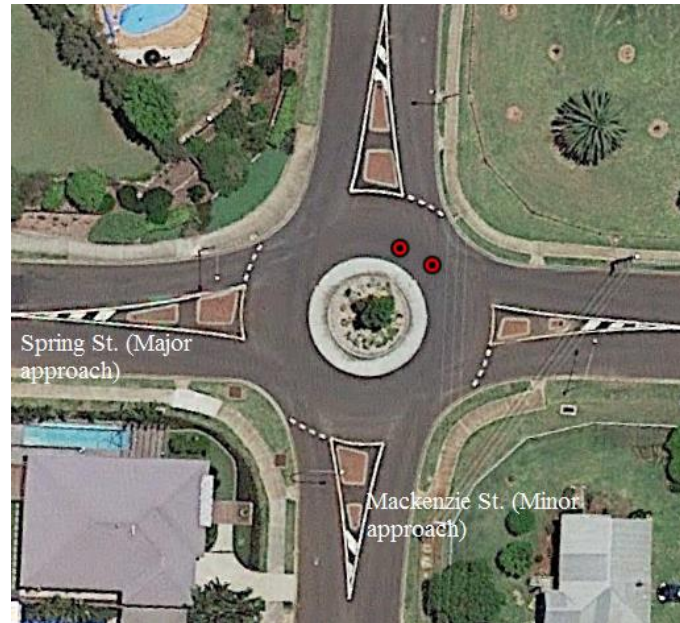
Figure 5.22 Roundabout R_SE2 between Spring Street and Mackenzie Street (Source: Aerial Image from Google Earth pro)
