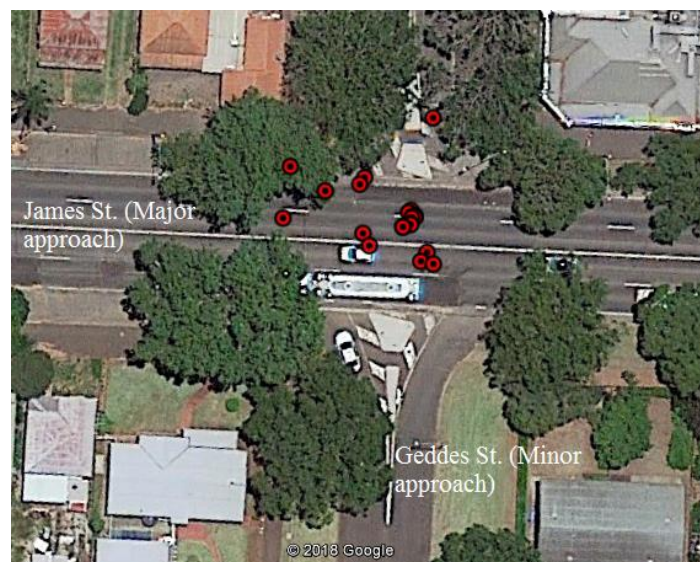
Figure 4.11 Intersection I_NE6 between James Street and Geddes Street Source: Aerial Image from Google Earth Pro
