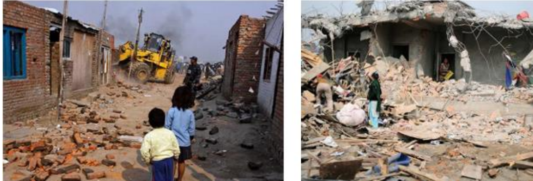
Figure 3-11: Bulldozing of informal settlement at Sankhamul Source:(Joshi, 2012)
