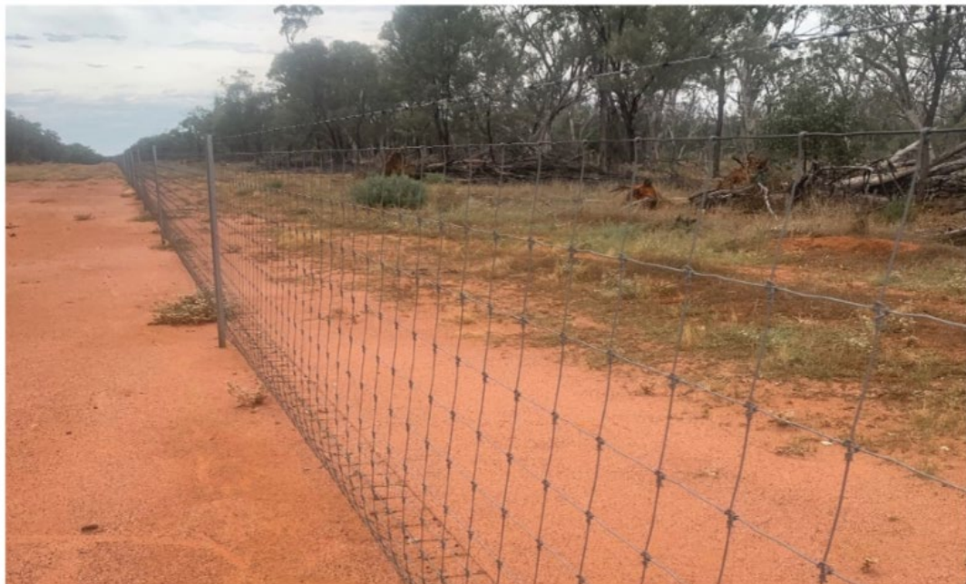
Figure 2.6 A typical section of dingo-proof exclusion fence (Source G. Castle 2021) .
