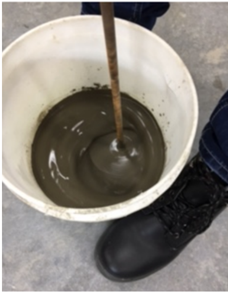
Figure 3.24: Grout preparation
