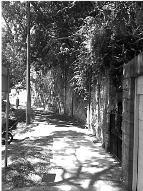
Figure 6: An example of a tall retaining wall on the opposite side of the pathway to the street verge. Image taken on a hazy day at 2:00pm local time, 21 st November 2019.
