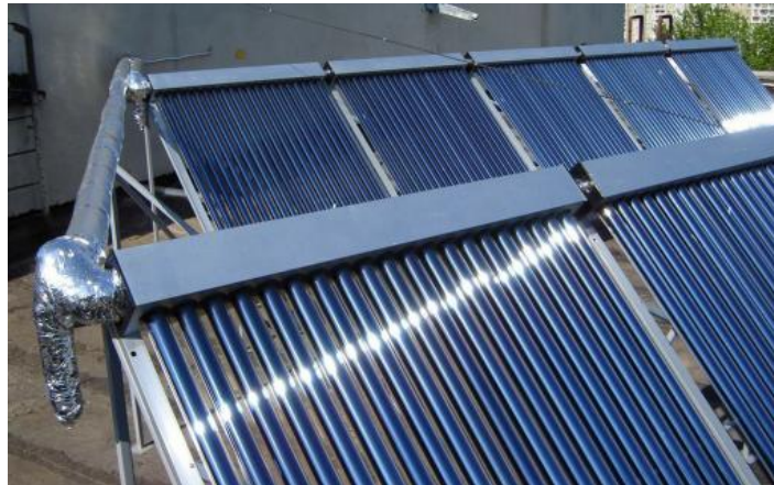
Figure 4: A sample ETC installation, (Source: Solar and wind energy, 2010)
