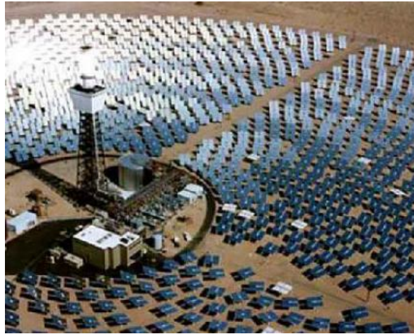
Figure 7: "Power Tower" and arrayed heliostats
