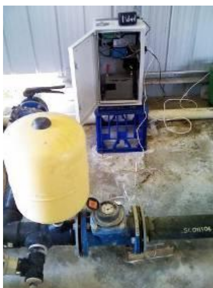
Figure 9. High frequency flow meter logging at an orchard near Gatton
