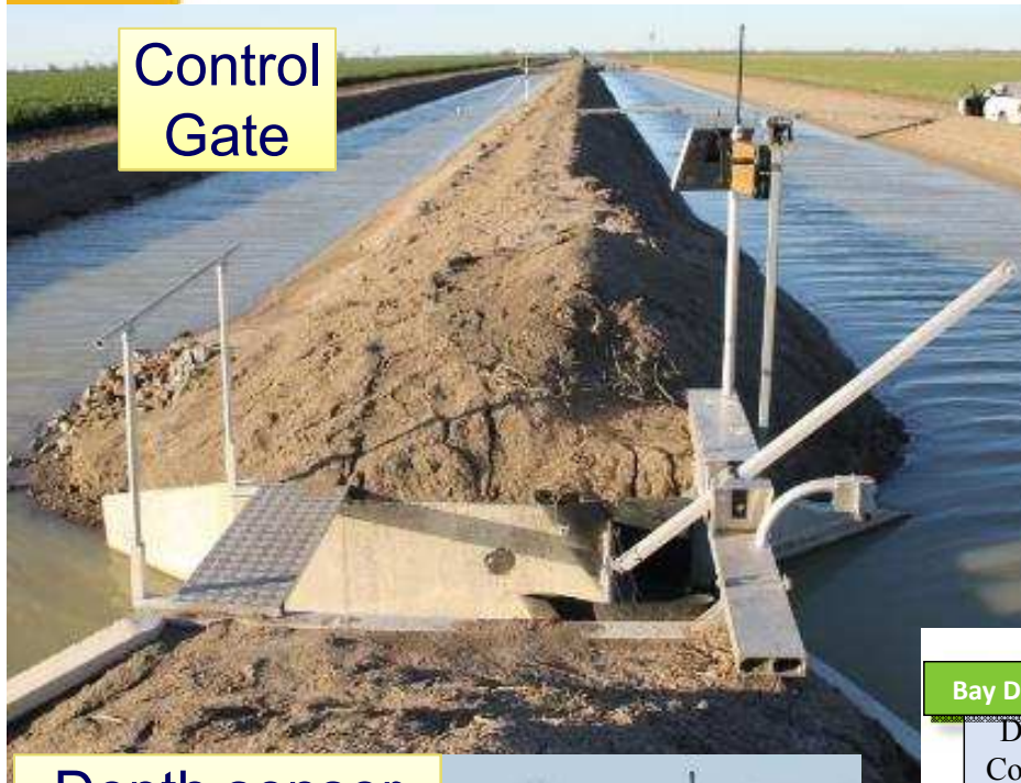
Depth sensor for flow meas. and control of channel system
