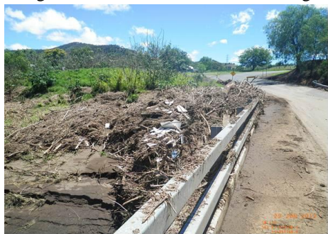
Damaged due to debris
