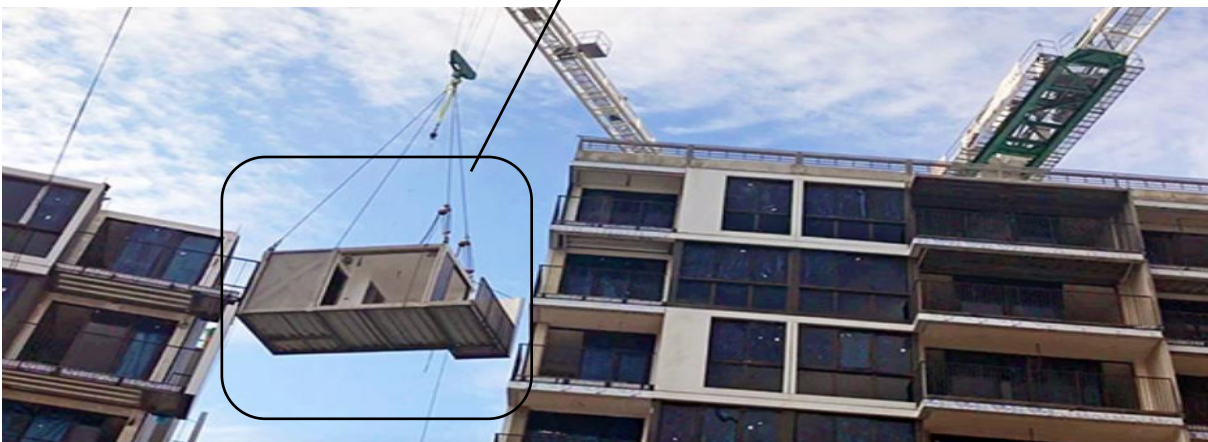
Figure A15.2 Modular Integration Construction Method (Courtesy Image from Hong Kong Government, 2022, 2023)
