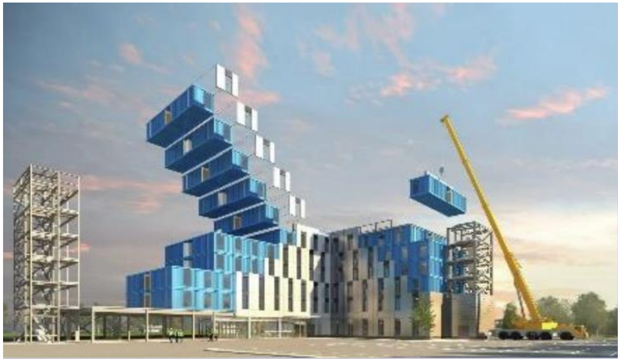
Figure A15.3 Modular Integration Construction Method (Chung and Chan, 2021)
