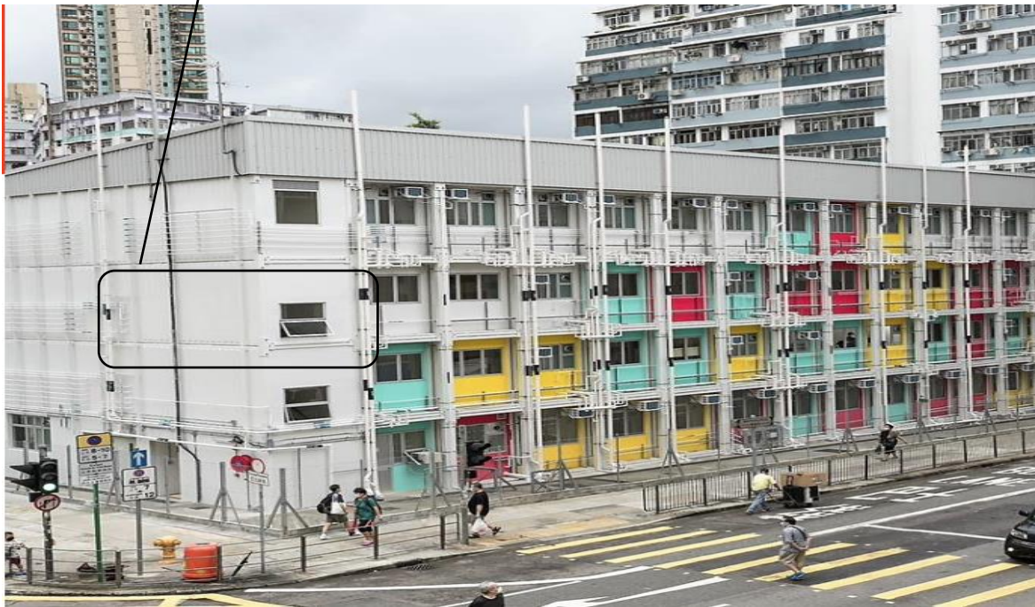
Figure A15.1 One Example of Modular Integration Construction (Hong Kong Government, 2022, 2023)
