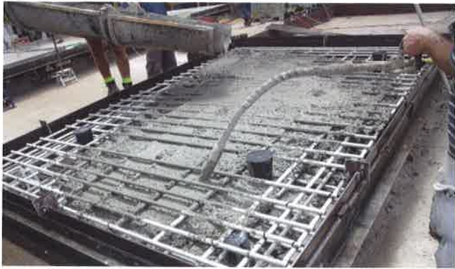
Figure 11: Wyndham jetty precast panels (left) and the jetty under construction (right).
