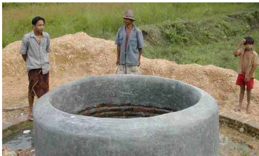
Figure 6.20 Shallow dug well in Lombok Tengah.
