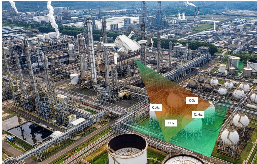
Figure 3. Equipped with specialised sensors to monitor hazardous environments, drones can detect odourless and colourless toxic gases.
