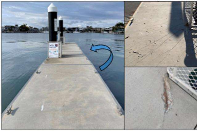
Fig. 1. Pontoon in wave action, torsional cracks and reinforcement corrosion.
