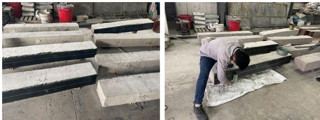
Fig. 2. Reinforcement with CFRP sheet for the bottom face of the beam.
