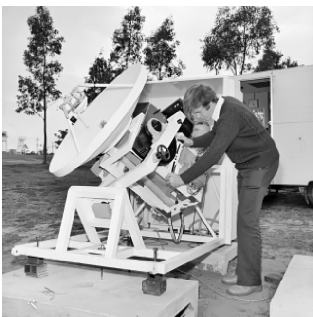
Figure 14. John Archer working on the 1-metre telescope, with which he, Norman Labrum and Christopher Smith observed the Sun at 3-mm from Stawell during the 1976 eclipse (Image Credit: CSIRO Radio Astronomy Image Archive).
