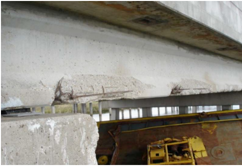
450 Figure1: Damage due to impact (Padgett et al. 2008)
