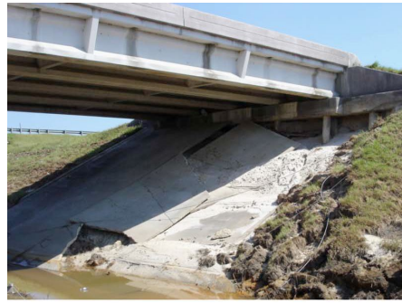
Figure 2: Damage caused by scouring (Padgett et al. 2008)
