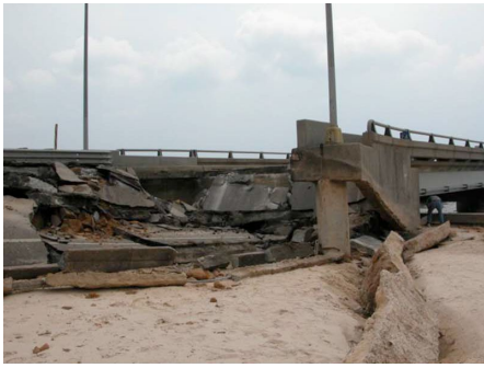
Figure 2: Damage caused by scouring (Padgett et al. 2008)
