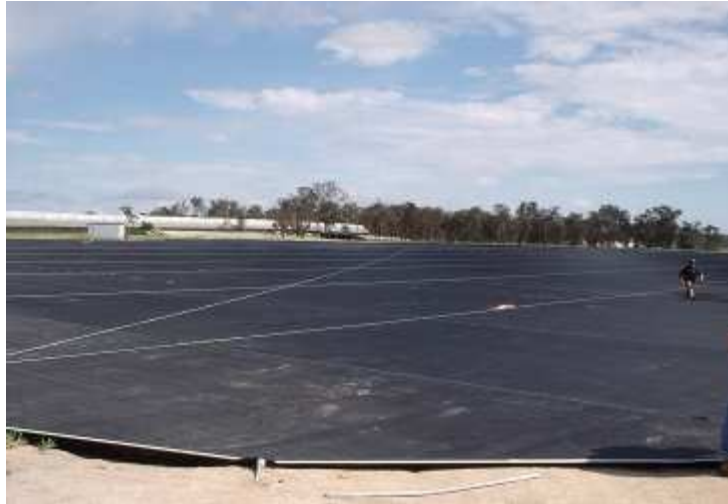
Figure 5: Shadecloth cover installed at Andreatta's Farm, Stanthorpe Qld
