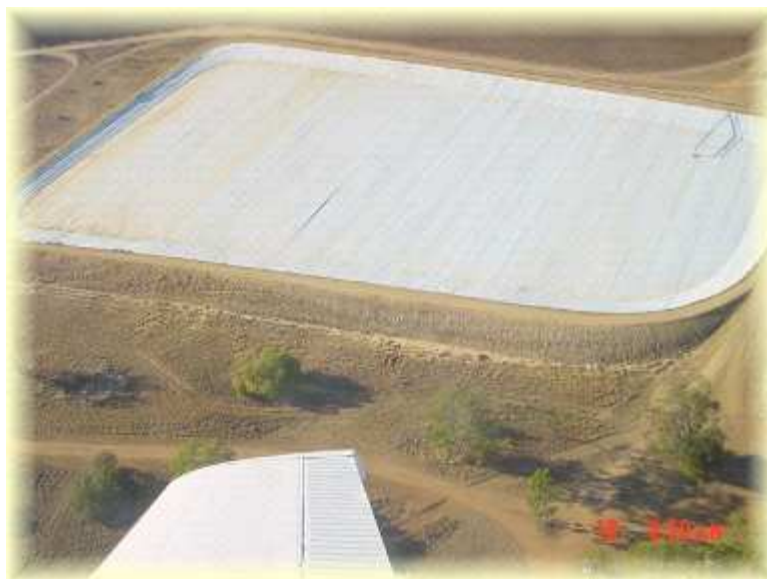
Figure 4: Plastic cover (E-VapCap®) newly installed at Moons Farm, St. George Qld
