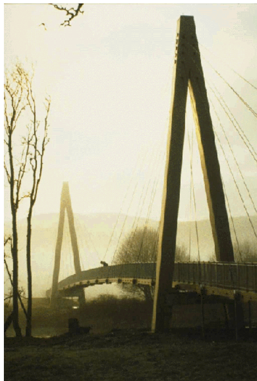
Figure 1.1 FRP pedestrian cable stay bridge across the River Tay in Aberfeldy, Scotland (Barbero 1998)
