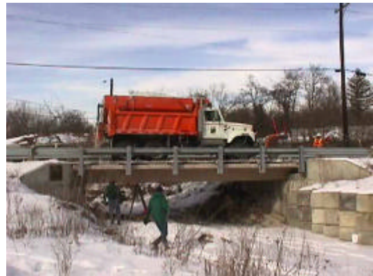
Figure 1.4 Vehicular bridge in the City of Hamilton, Butler County, Ohio (iCivil)
