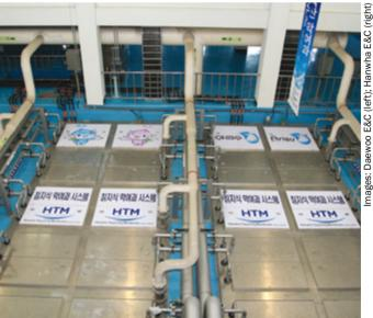
Yeongdeungpo waterworks: the DIMS pressured membrane (left) and HTM submerged membrane (right)
