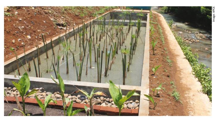
One of the constructed wetlands used to improve domestic wastewater treatment
