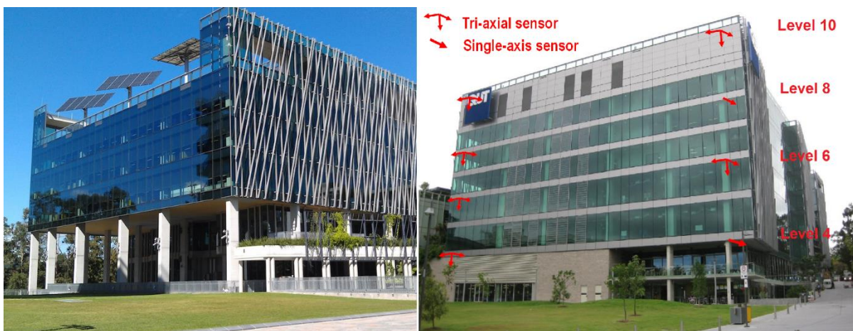
Figure 2 P block building: front corner view (left) and side view with sensor positions (right)
