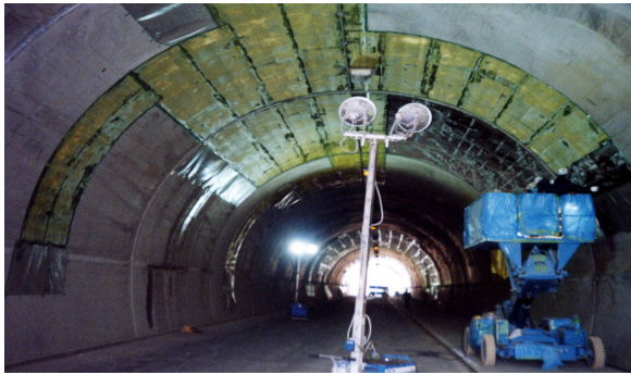
Figure 7. Retrofitting tunnel
