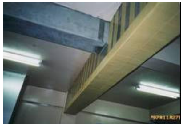
(b) Retrofitting beam
