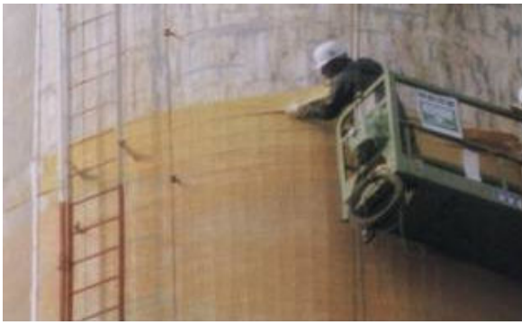
Figure 6. Retrofitting chimney
