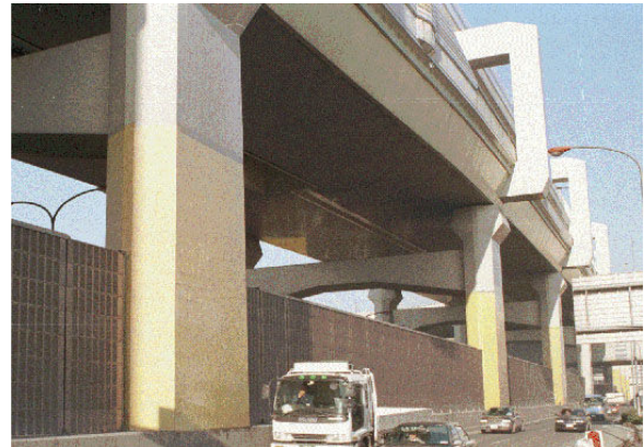
Figure 4. RC bridge piers retrofitted by AFRP sheets
