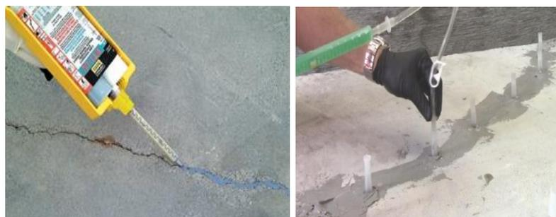
**Figure 2.1:** Concrete crack repair- epoxy resin injection ([www.strongtie.com.au](http://www.strongtie.com.au))
