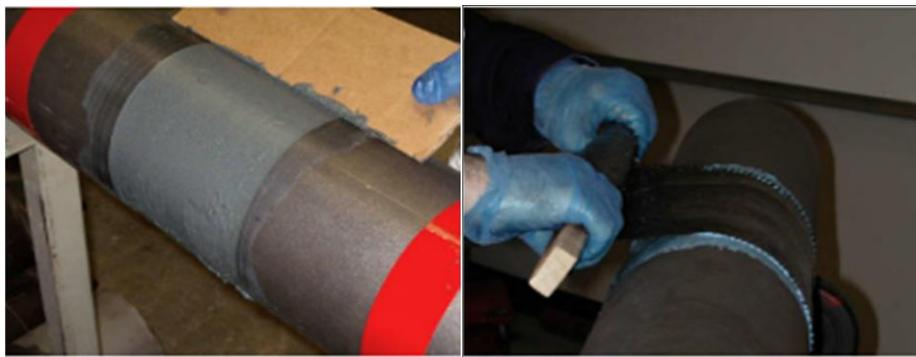
**Figure 2.3.** Pipe exterior repair using infill and flexible wrap, filling defect with putty and wrapping epoxy wetted carbon fabric around the defect (Duell et al., 2008)
