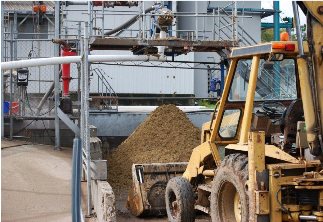
Figure 22 - Paunch on site at CA passes from the screw press to fall into a pile in the cement holding area.
