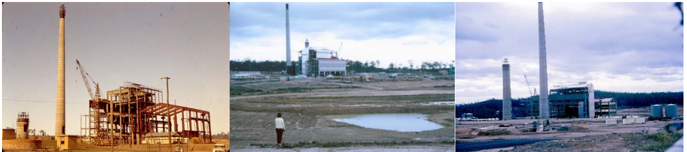
Figure 31 (a–c): (left) Swanbank A under construction 1965 and (centre & right) 1965 & c1966. (Picture Ipswich).
