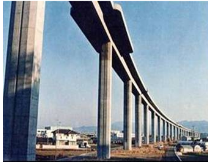
(a) Shigenobu river bridge, Japan
