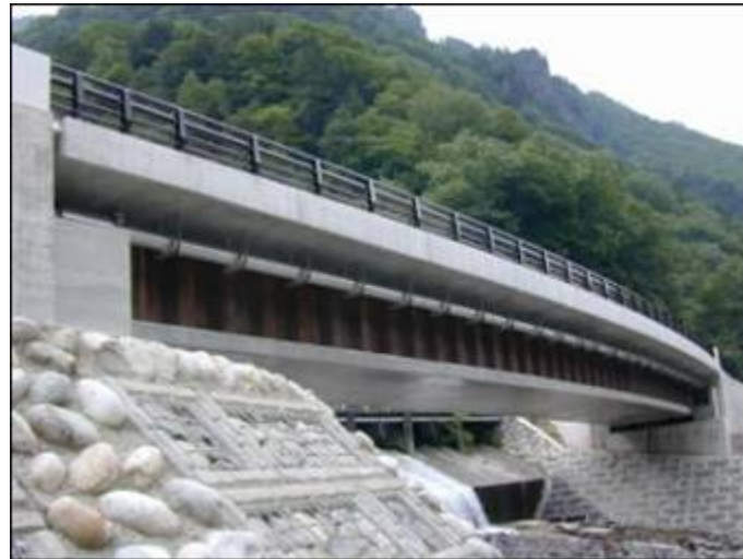
(a) Completed view of Shirasawa bridge, Japan
