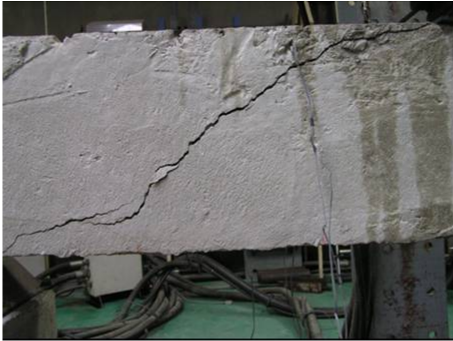
Figure 4.19. Failure of control beam ECL31
