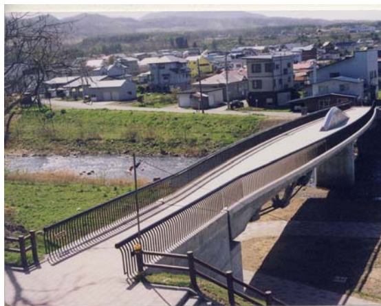
Figure 2.4. Pedestrian bridge with large eccentricity post-tensioning tendons Source: DPS Bridge Works, Tokyo, Japan
