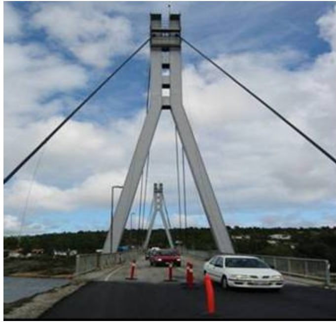
Figure 2.9. Rehabilitation with lightweight concrete – Puttesund Bridge, Norway Source: http://gallery.kak.net/
