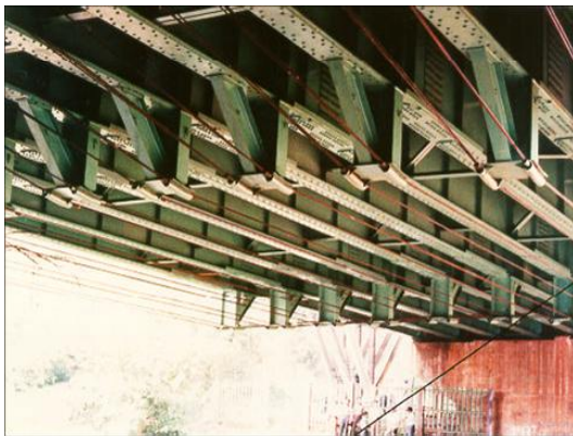
(a) Condet bridge, Indonesia
