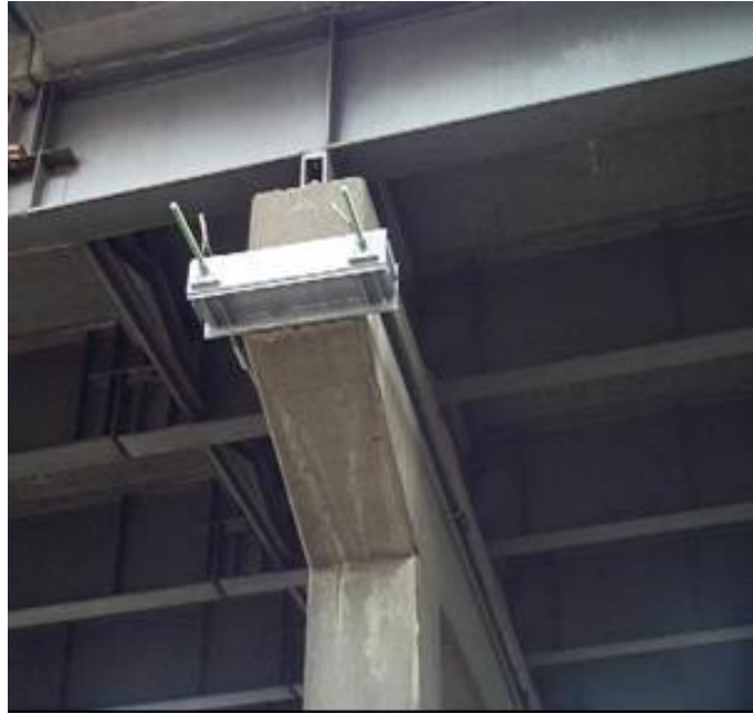
a) Morrison bridges headstock, USA Source: http://www.co.multnomah.or.us/
