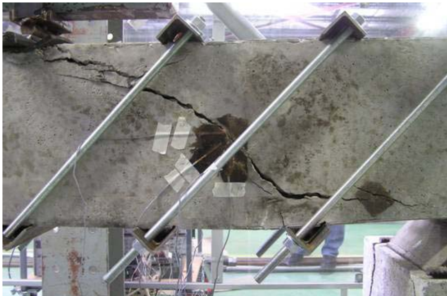
Figure 4.1. Failure due to concrete crushing
