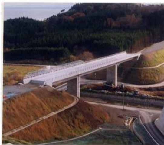
(a) Shirarika river bridge made of HLA concrete
