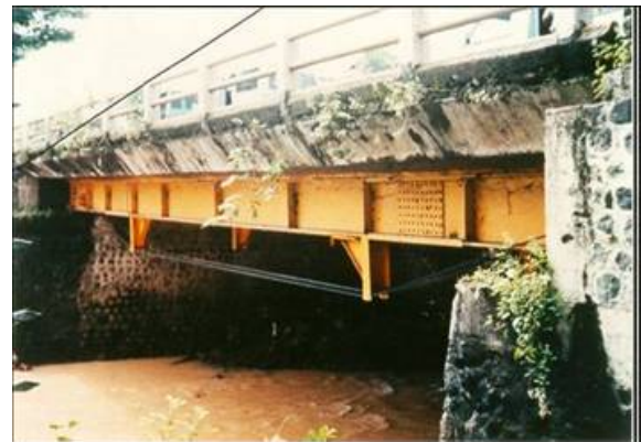
(b) Kemlaka Gede bridge, Indonesia
