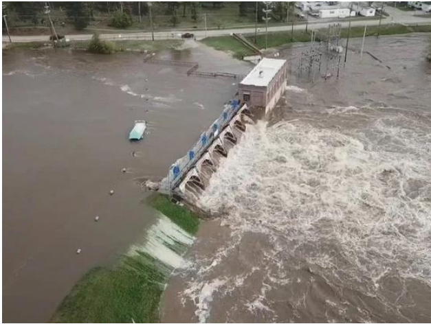
a) Failure of Sanford Dam-Michigan, USA (WION Web Team, 2020)
