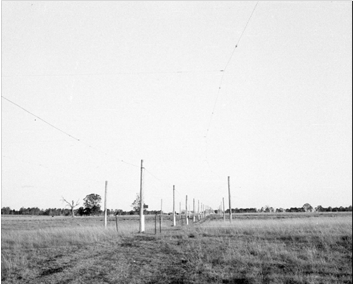
Figure 16: A view looking north along the N–S arm of the Shain Cross, showing the central line of poles that carried the coaxial feeder cable, and the adjacent poles that supported the dipoles (courtesy: CSIRO RAIA 5753-4 cropped).
