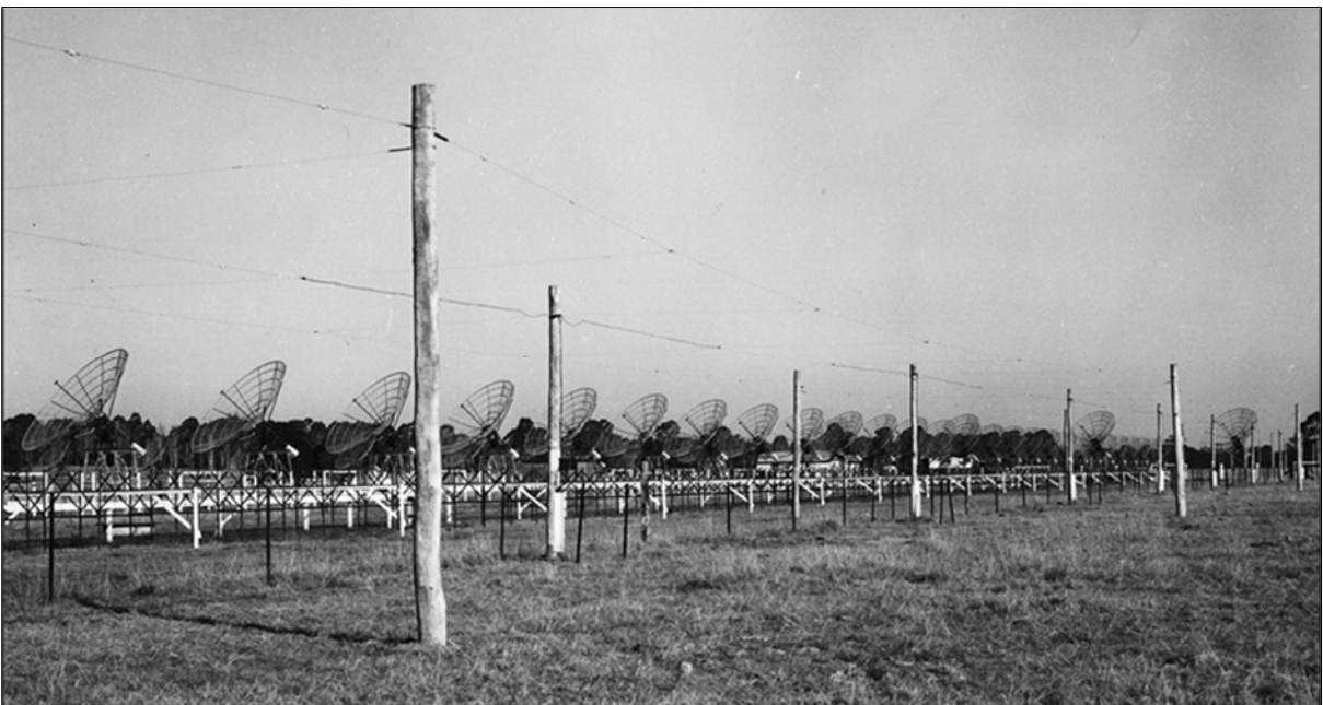
Figure 17: A view looking south along the N–S arm of the Shain Cross, showing part of the adjacent N–S arm of the 85.5 MHz Mills Cross and parabolas in the N–S arm and part of the E–W arm of the 1400 MHz Chris Cross solar grating array (courtesy: CSIRO, RAIA 5192-9).
