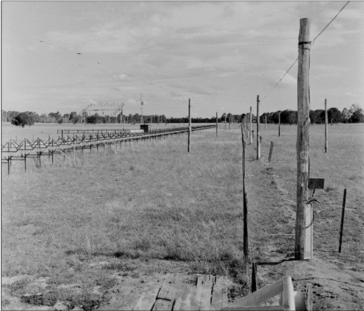
Figure 18: A view looking south along the N–S arm of the Shain Cross, showing part of the adjacent N–S arm of the 85.5 MHz Mills Cross. Beyond it, to the left, is a broadside antenna that was used with a similar antenna at nearby Badgerys Creek field station to investigate Hydra-A and the sizes of some of the Mills Cross discrete sources (courtesy: CSIRO, RAIA B3868-19).
