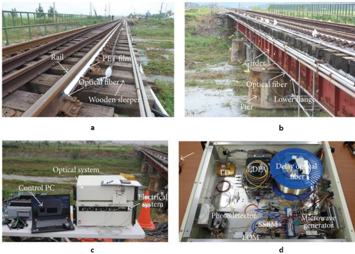
Figure 2.9: Monitoring site at Cheong-ri Bridge [117] (a) Optical fibre mounted on the outer surface of the rail; (b) mounted on the lower flange of the girder; (c) DOFS system based on BOCDA method; (d) configuration of the optical system
