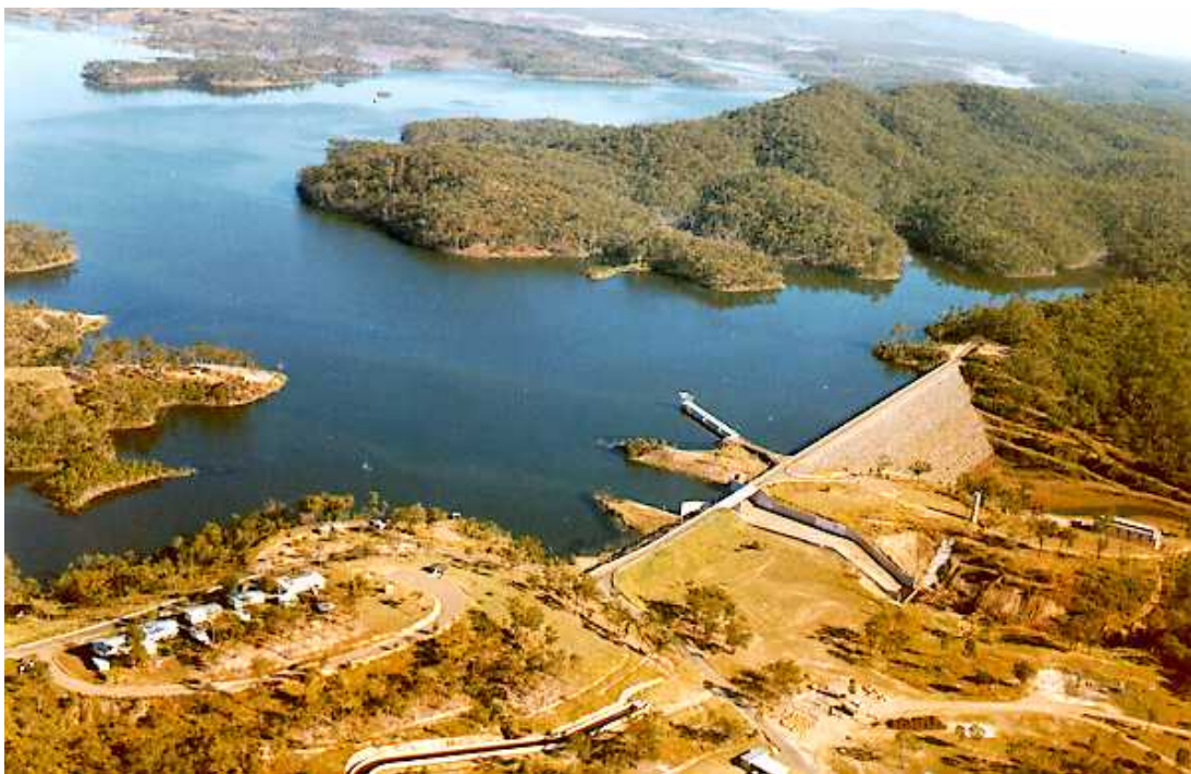
Figure 1-1 Fred Haigh Dam
