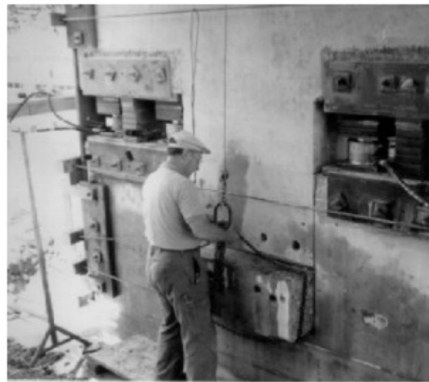
b) Pier settlement using hydraulic jacks
