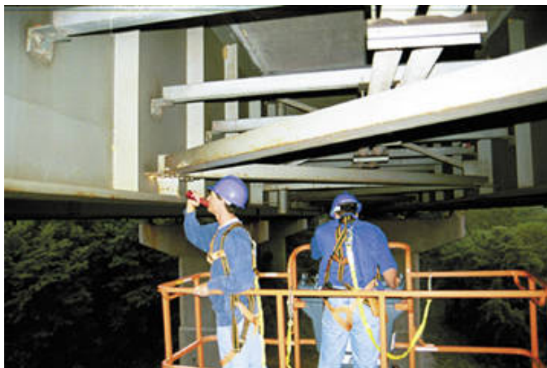
Figure 4 Visual inspection on a bridge girder (64)
