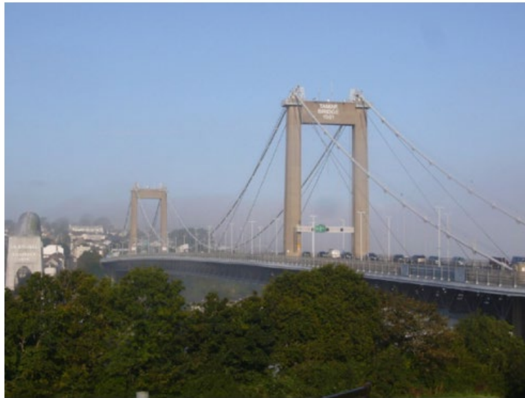
Figure 14 The Tamar suspended bridge
