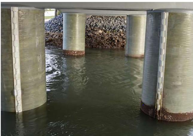
Fig. 17. Bridge piles repaired with FRP jacket [166].
