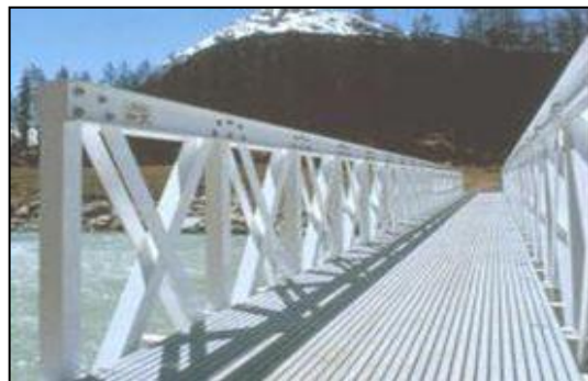
Figure 2.10. The all FRP composite Pontresina bridge (Keller et al. 2007)
