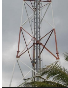
Figure 1.3 Space trusses (steel) in telecommunication tower
