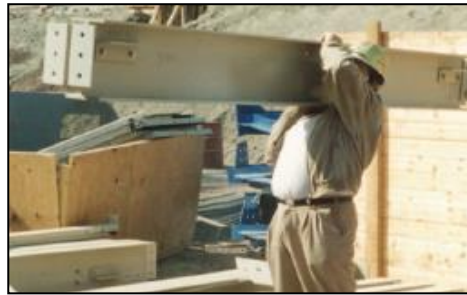
Figure 2.4. Lightweight pultruded FRP beam structures ( www.strongwell.com/literature )
