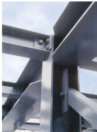
Figure 1.4 Example of frame bolted connections ( www.strongwell.com/literature )
