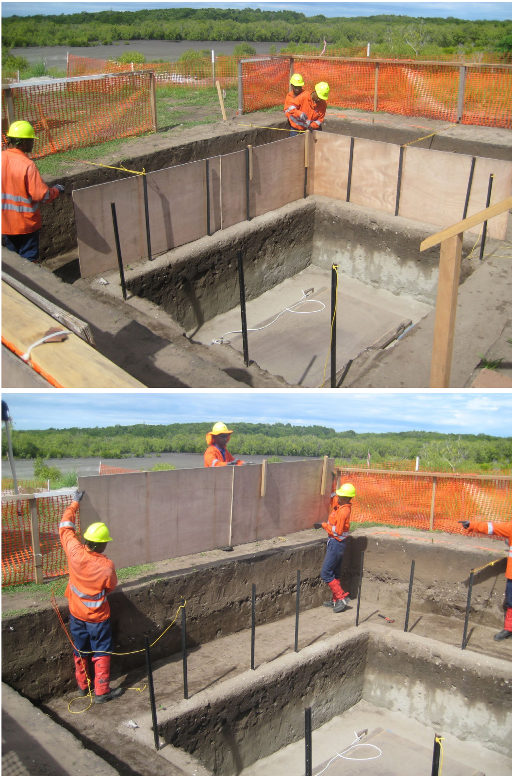
Figure 2.11. Removing shoring after excavation of the outer ring of excavation squares, Tanamu 1. The central trench (Squares A and B, bottom-right of photo) is covered by a wooden lid.
