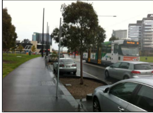
Figure 2.2 - Bioretention street trees (obtained from guide to the cost of maintaining bioretention basin prepared by Water by Design)
