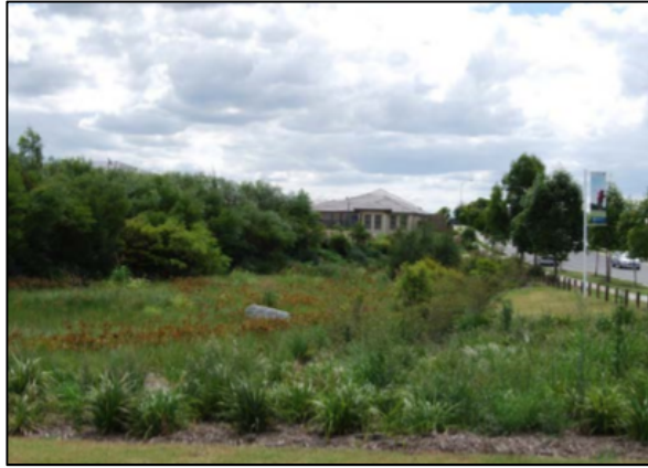
Figure 2.4 - Precinct scale bioretention basins (obtained from guide to the cost of maintaining bioretention basin prepared by Water by Design)
