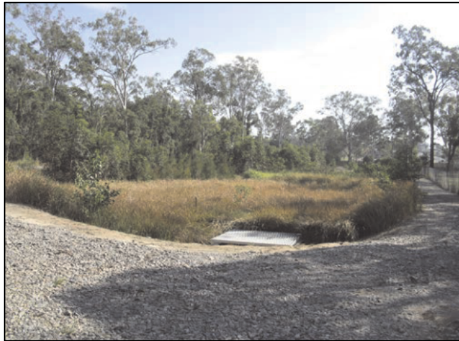
Figure 2.5 - Large biorientation basin (obtained from guide to the cost of maintaining bioretention basin prepared by Water by Design)
