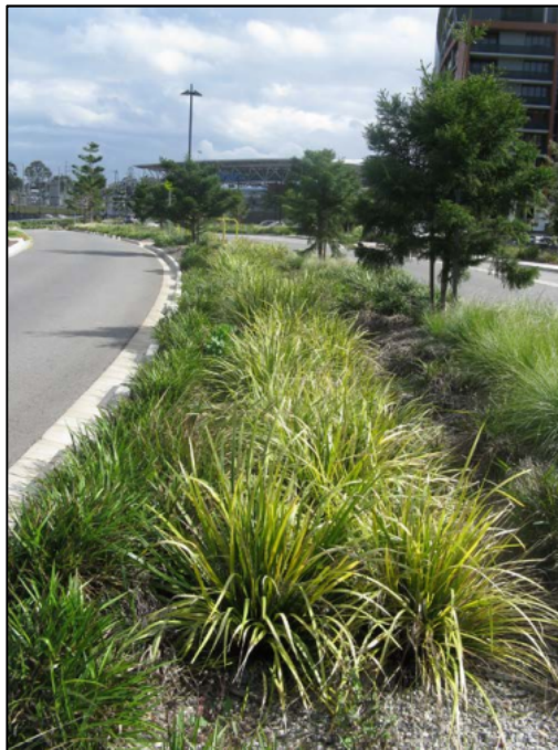
Figure 2.3 – A streetscape bioretention system (obtained from guide to the cost of maintaining bioretention basin prepared by Water by Design)
